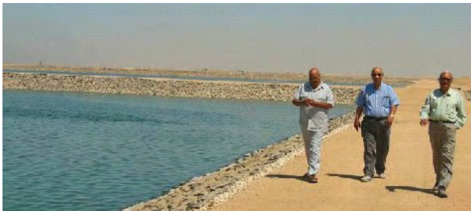
Figure 8 Maturation Pond Adjacent to Demonstration Site
