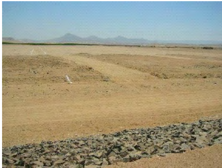
Figure 4 Demonstration Site Looking East (dike structure in the foreground)
